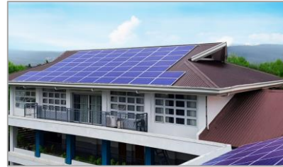
St Mary University Philippines 219 kWp, 2017
