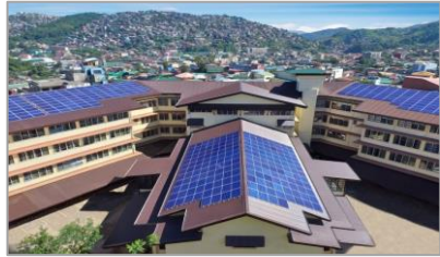
St Louis University Philippines 243kWp, 2018
