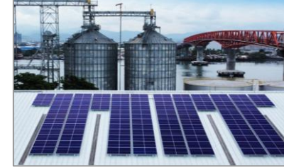
Mactan Grains Terminal Inc. Philippines 55 kWp, 2023
