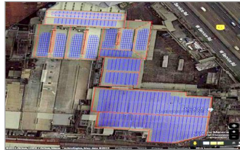
CDO Foodsphere Inc. Philippines 955.84 kWp, March 2024
