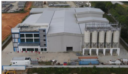
Joe Green Precast Malaysia 1,200 kWp, March 2024
